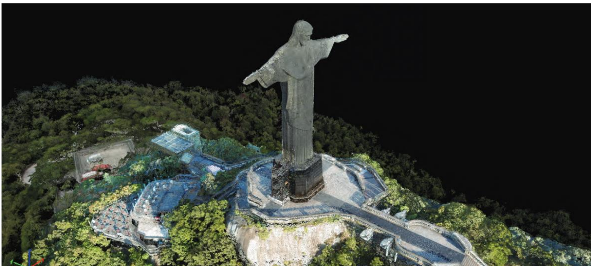
Point Cloud of statue and surrounding area
