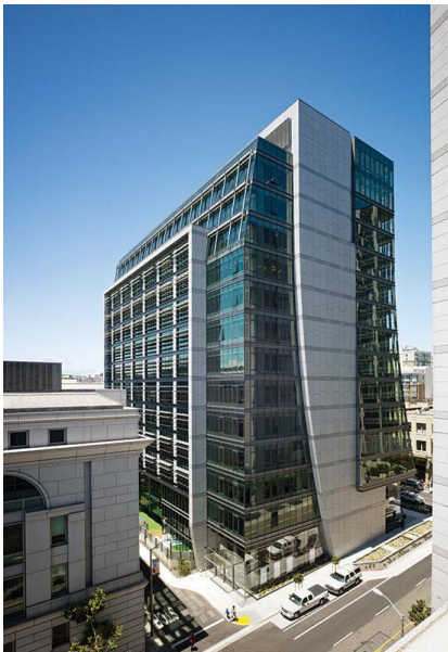
Utility operations building in San Francisco, CA
