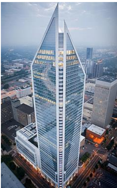
Duke Energy Center, N. Carolina, Virginia
