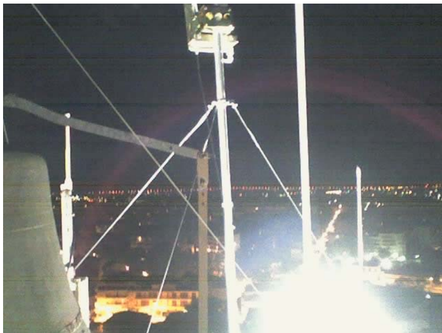
Figure : WiMAX CPE installed in Trikala, Greece
